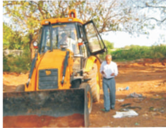
Active disposal area located at Karuvadikuppa village, Puducherry
