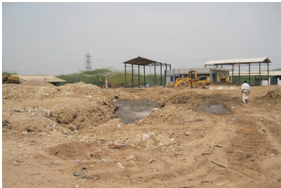
Okhla, New Delhi Land fill site
