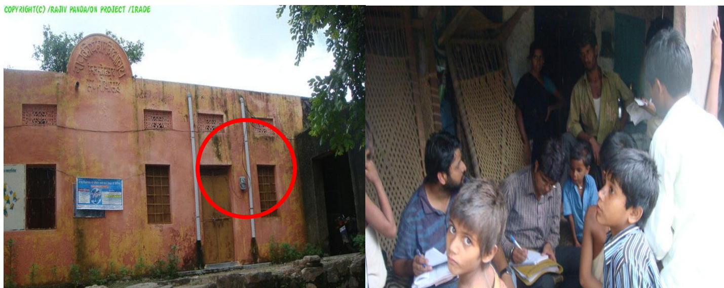
Figure 19 Left Photo- one of the electrified school in Rajasthan, Meter installed in the School, Right Photo- School children are being asked about the benefit of the electricity.
