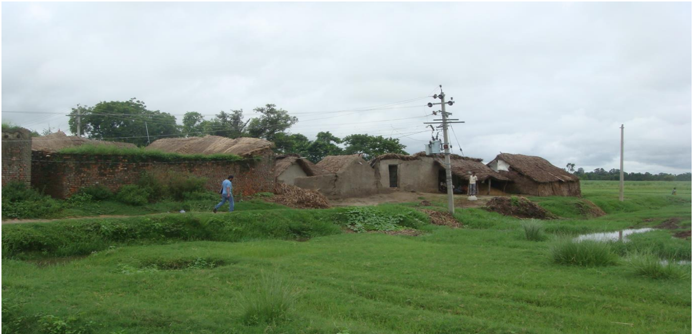
Figure 1 Last Mile Household is being Surveyed by IRADe- Remote villages/households has been electrified, bringing access to power
