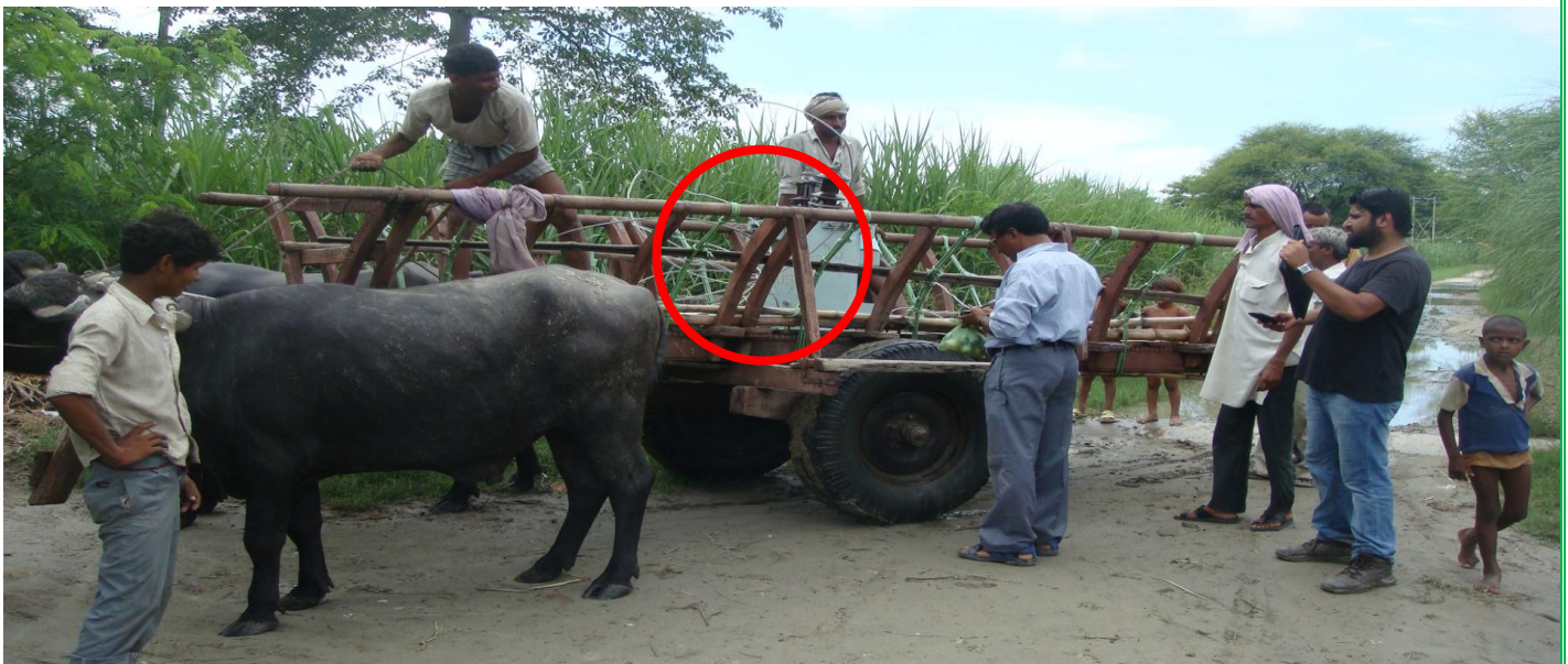
Figure 20 shifting of transformer by villagers without the proper approval from the Discom.
