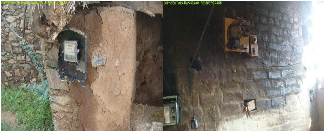
Figure 6 Left Photo- Meter damaged, right Photo- Meter installed in the Kitchen of the House and has damaged the meter.
