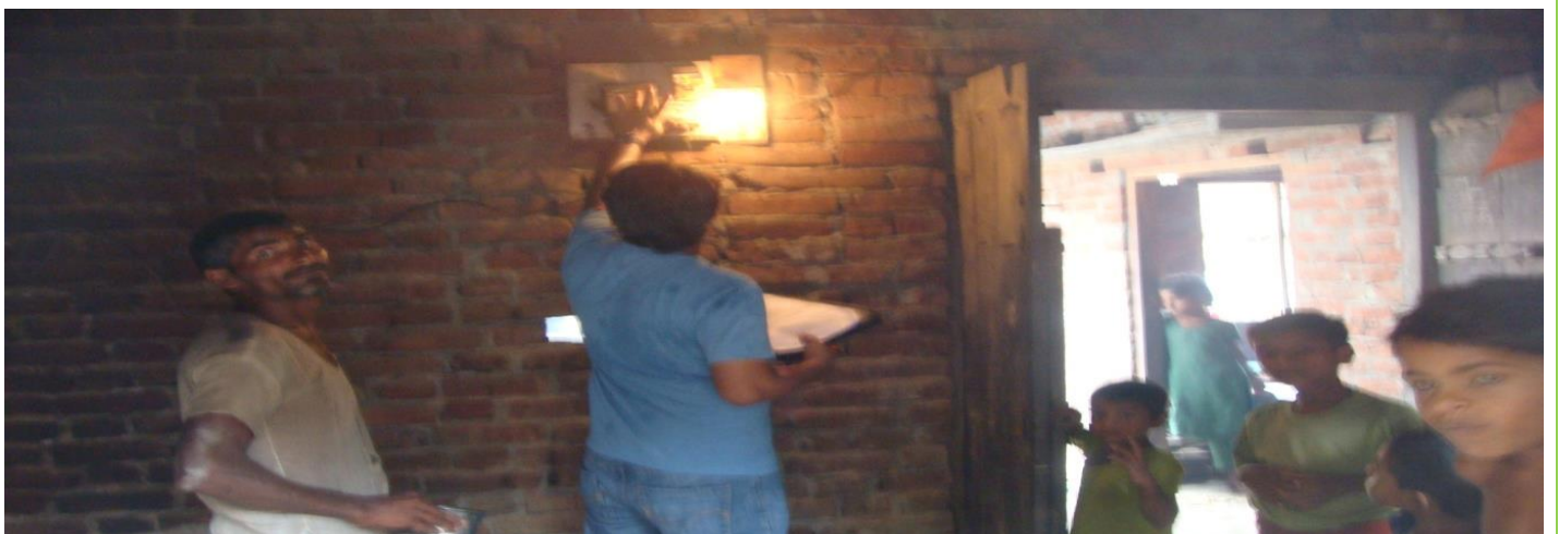
Figure 22 Meter Condition is being checked by the IRADe team member
