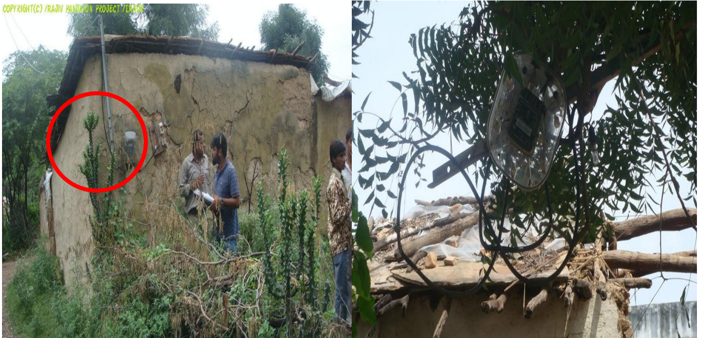
Figure 7 Meter installed in the back side of the House in the open, leading to damage of the meter, Right Photo- Meter Installed in a Tree.
