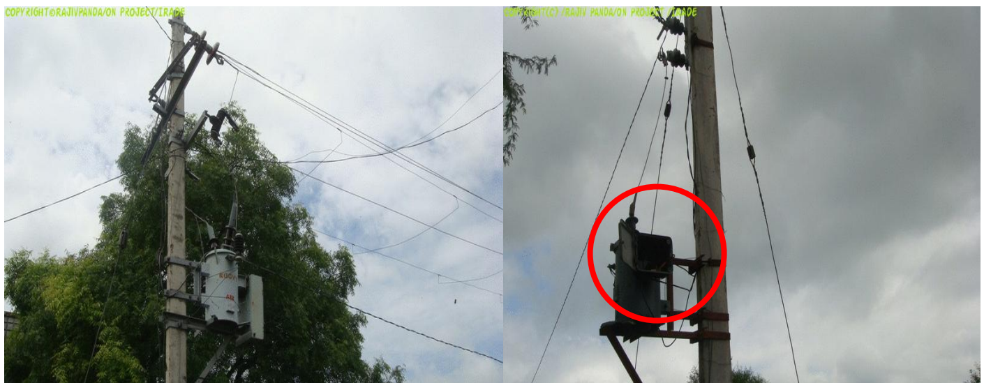
Figure 5 left Photo - A transformer damaged, Right Photo- Transformer protective device are removed by the villagers due to the frequent tripping due to overloading.
