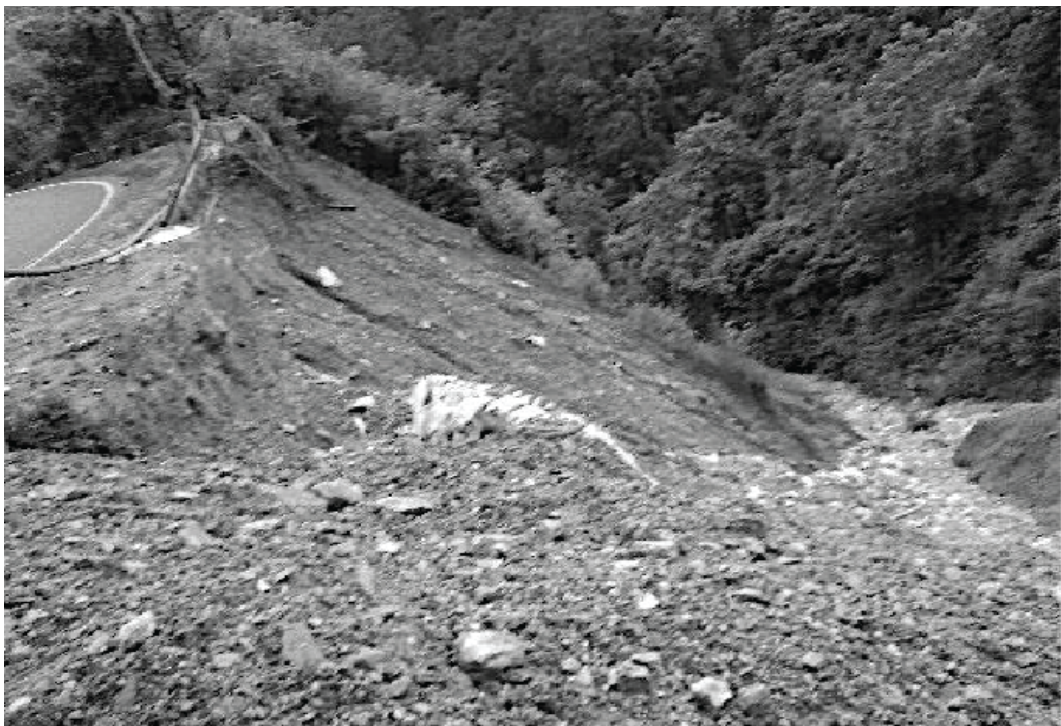
Figure 5: Landslide Along Guwahati-Shillong Road Near Ryndang Brier, Shillong (25° 39.107' N and 91° 53.890' E)
