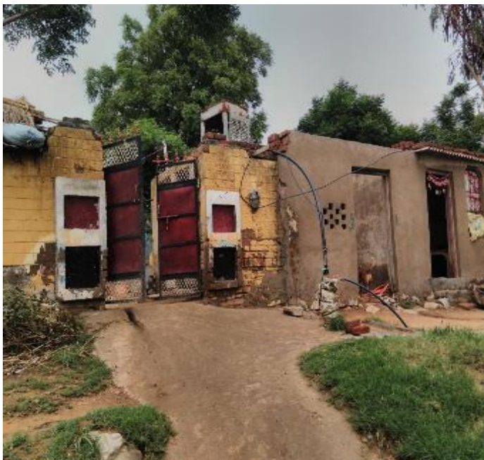
Electricity meter in a rural surveyed HH
