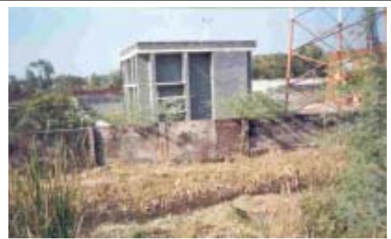
Photo 4.6: House made of fly ash bricks inside IFFCO. Plant.
