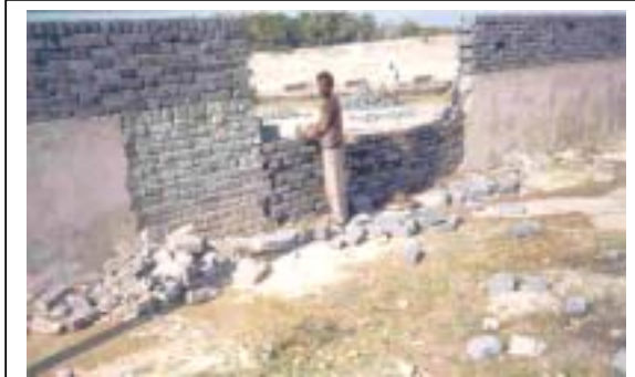
Photo 4.5: Construction of boundary wall using fly ash bricks inside IFFCO, Plant.
