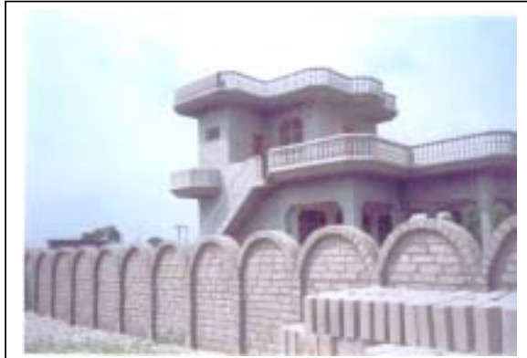
Photo 5.1b: Fly Ash Brick House, Constructed in 1998 by Ganga Brick Factory, Masoori, Ghaziabad.
