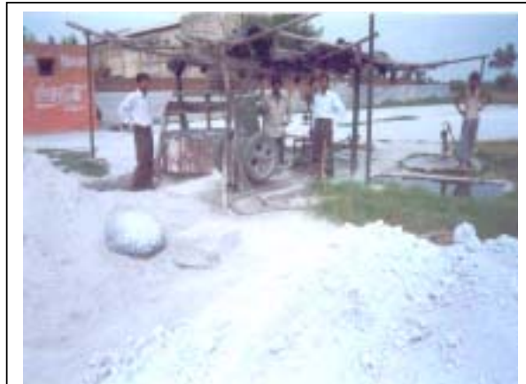
Photo 5.2: Mixer Machine with gypsum and fly ash.
