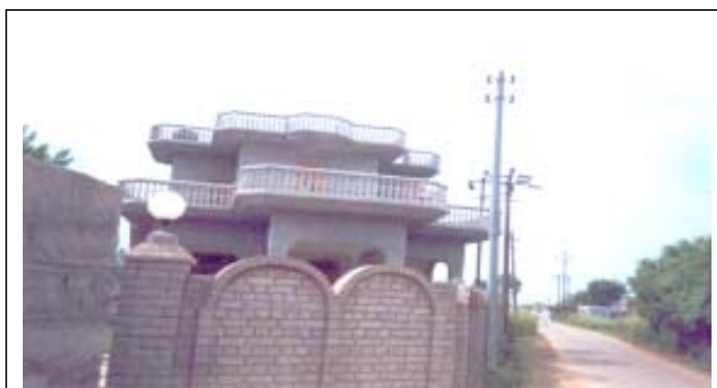
Photo 5.1a: Fly Ash Brick House, Constructed in 1998 by Ganga Brick Factory, Masoori, Ghaziabad.
