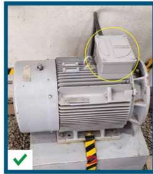
Motor terminal box in open and closed condition.
