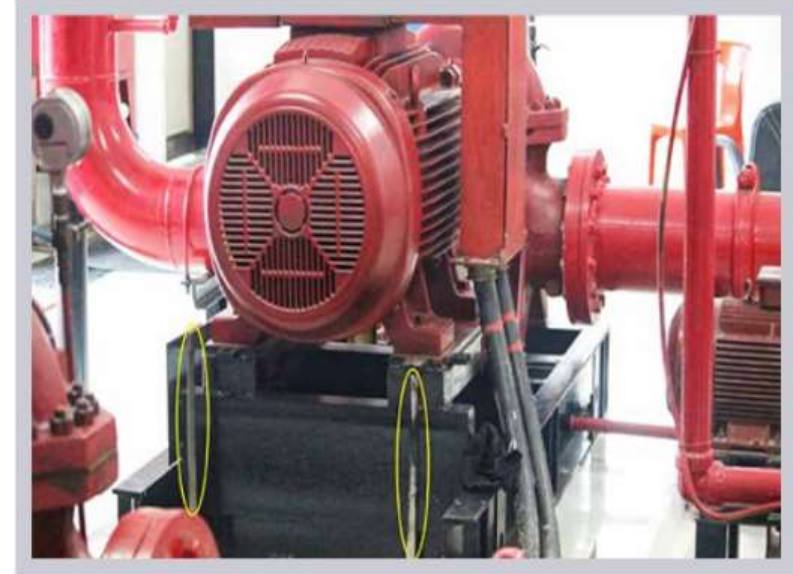
Motor double earthing
