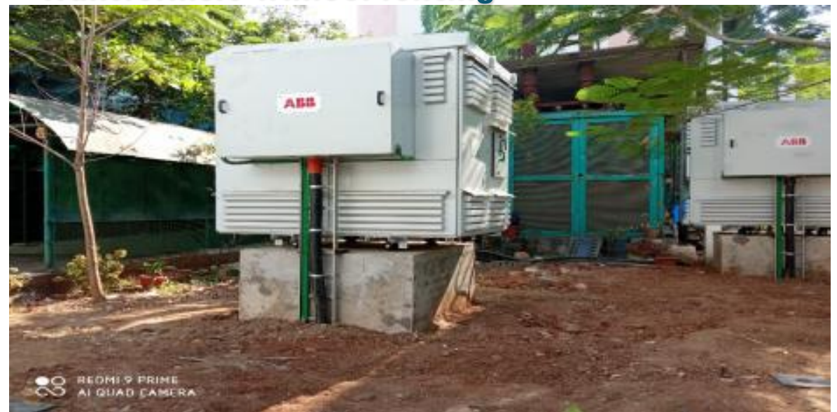
Transformers without fencing
