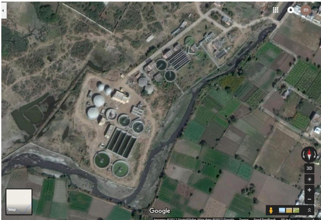
Google Image of under construction 60 MLD(40+20 MLD) STP at Ajmer
